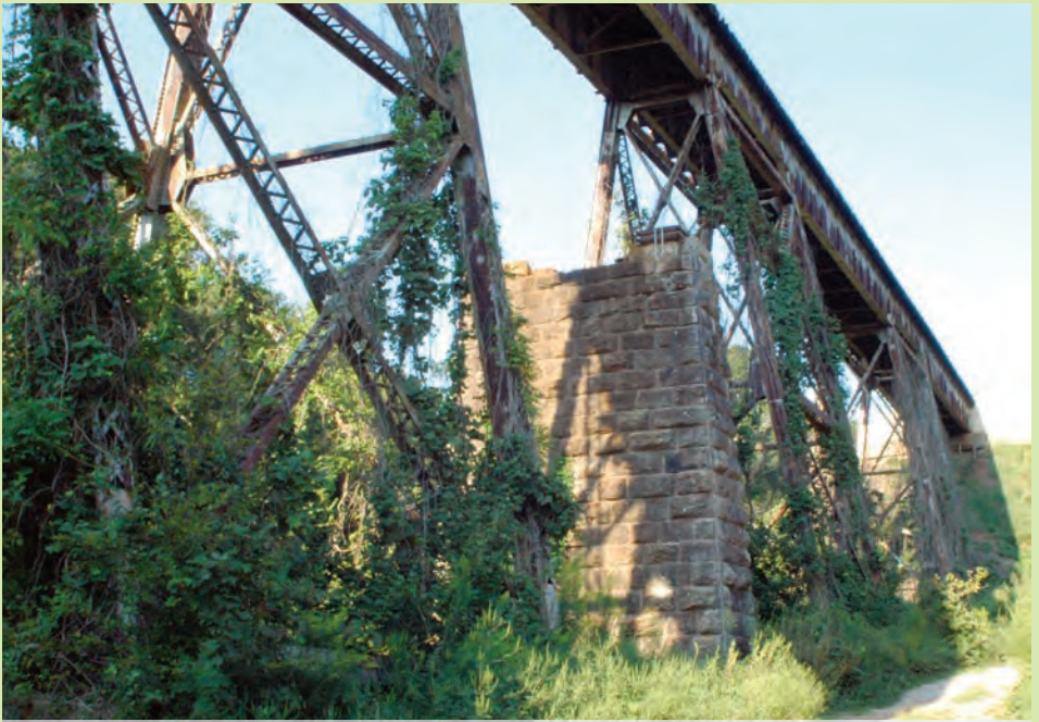
This stone abutment is still visible from the original bridge which was burned by General Sherman in 1864 on his March to the Sea. Photo: GWF
